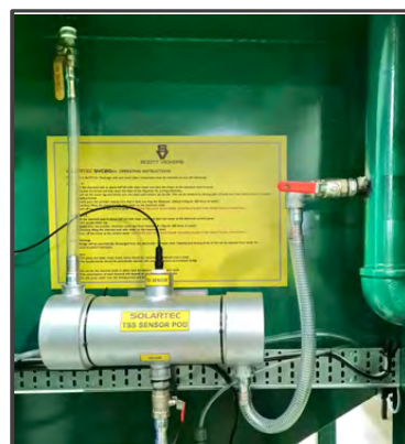
TSS SENSOR POD An alternative to the IBC TANK
